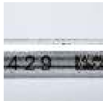
Fuel supply pipe code
